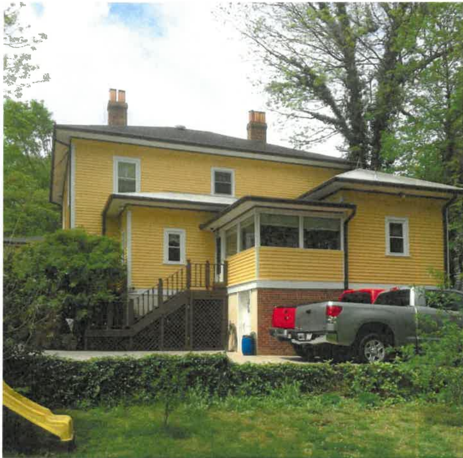
East (rear) facade
