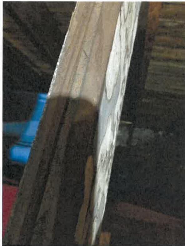
Attic beam in Henry Robins house; material salvaged from Marsh house shows Wallpaper from earlier era.
